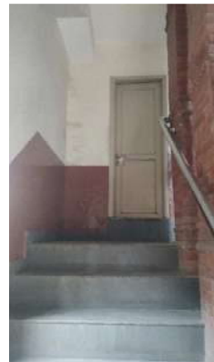
Staircase and toilets in landing area
