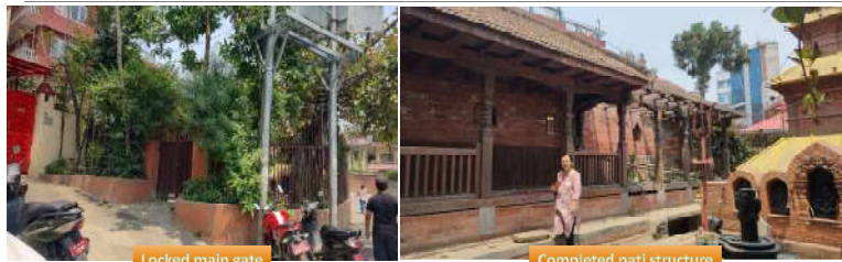
Locked main gate
