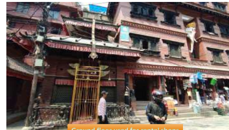
Ground floor used for rental shops
