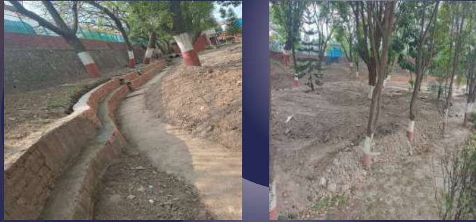
Beautification work at Sabhagriya Premises
