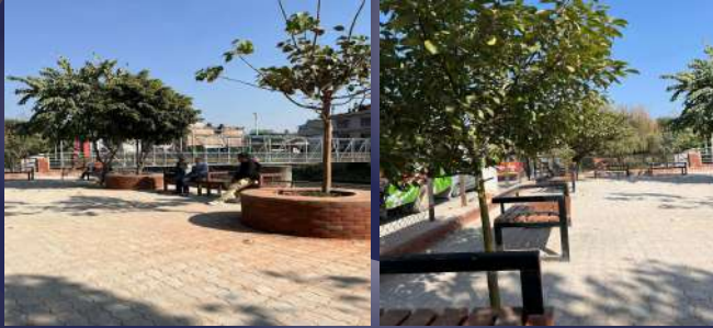
River and Road Beautification Works
