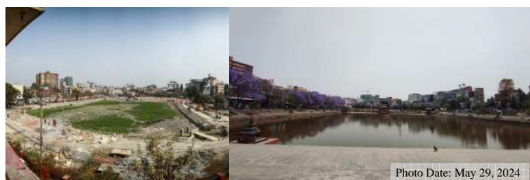
Kamal Pokhari during Construction
