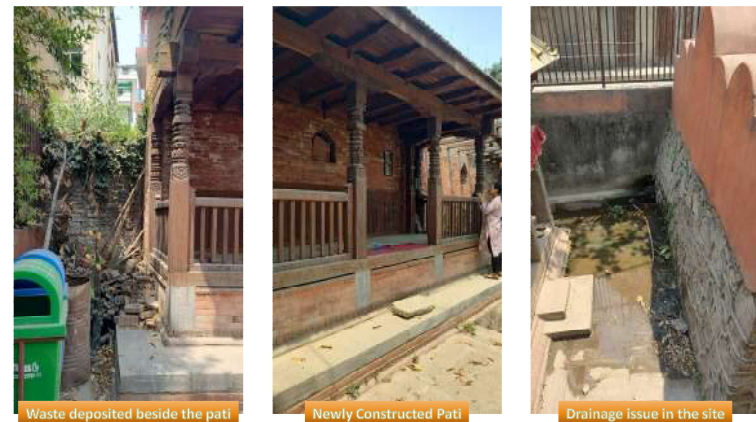
Waste deposited beside the pati
