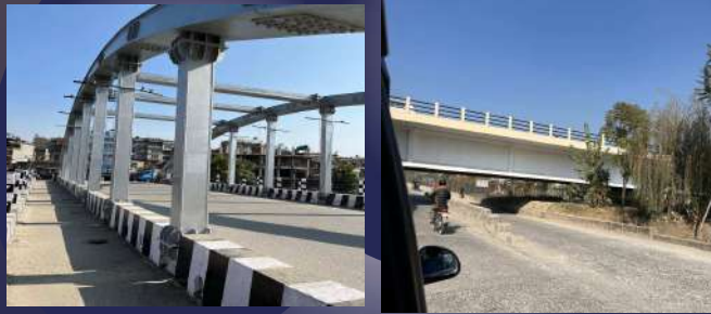
Painting Works(Bridge Painting, Pole Painting ,Tree Painting)
