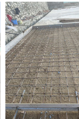
Concrete work at Transfer station.
